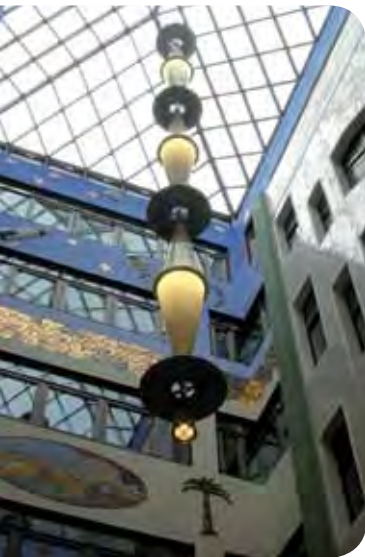
Shopping Arcade Renovation, Leipzig, Germany
