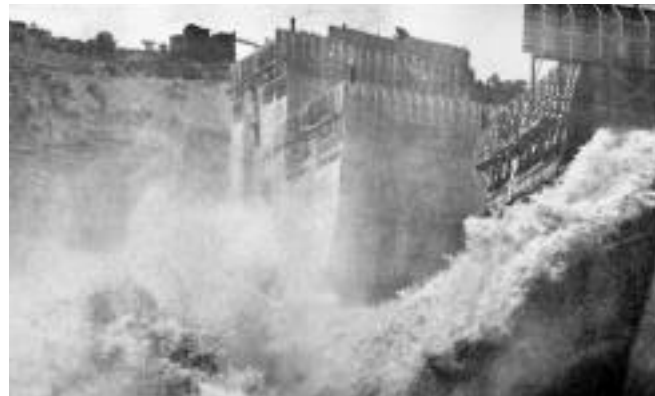
Figure 5.4. Zambesi River in full flood through Kariba worksite. Water flows of over 500,000 cubic feet per second were recorded.
