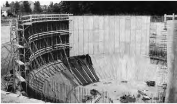
Figure 2.11 Seasonal storage tank under construction, Friedrichshafen. (Courtesy Renewable Energy World .)
