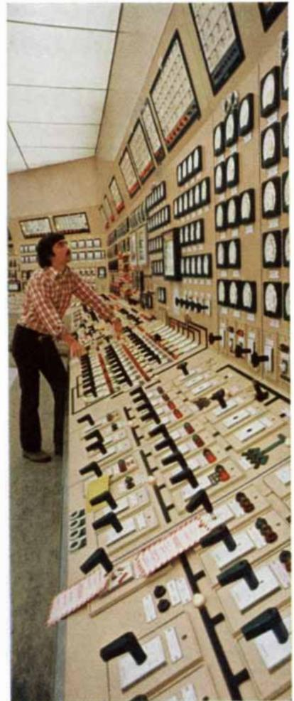
*In the control room of Zion Station, an operator monitors the voltage regulator on a 1,040 megawatt generator.*
