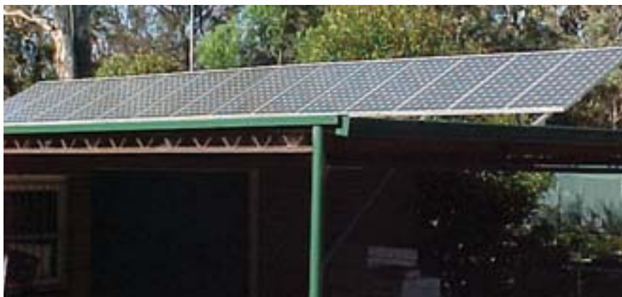
Solar panels on the Hornsby Community Nursery
