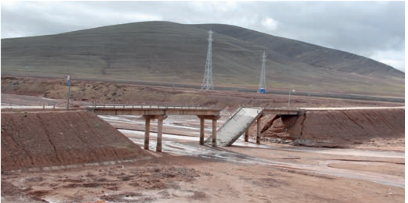
Figure 18: Permafrost thawing near the base of the support pillars caused this bridge on Qinghai-Xizang Highway in Tibet to collapse (photo: Tingjun Zhang).
